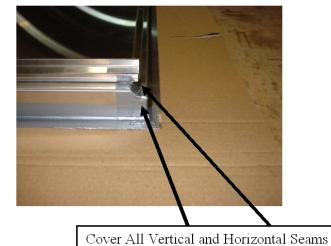
Apply Silicone Caulk Around entire flange (4) sides for final installation
